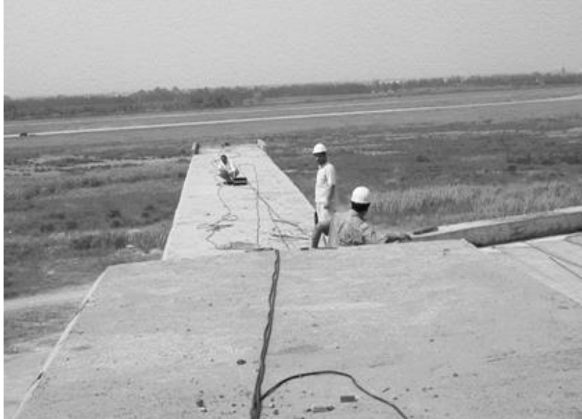
Figure 5: Ambient vibrations testing on the cell-box girder.
