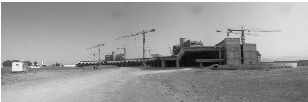
Figure 3: General view of the actual construction.
