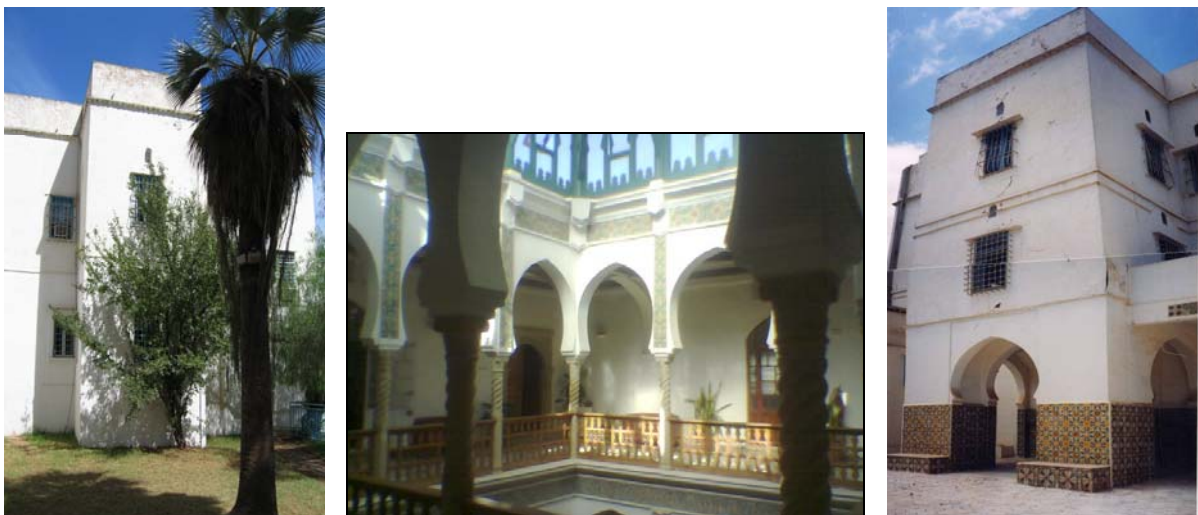
Figure 3. Exterior and interior views of the building
