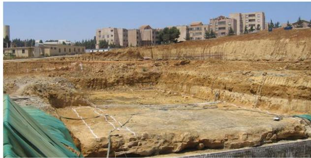
**Figure 3.** Soil conditions under the strong floor and reaction wall system during excavation on site
