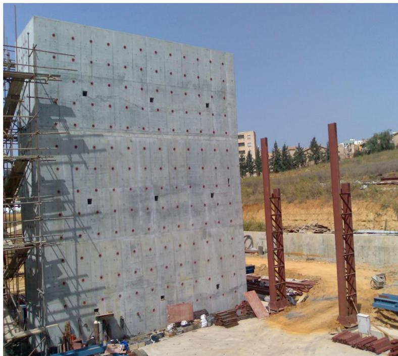
**Figure 1.** Global view of the reaction wall during the construction phase
